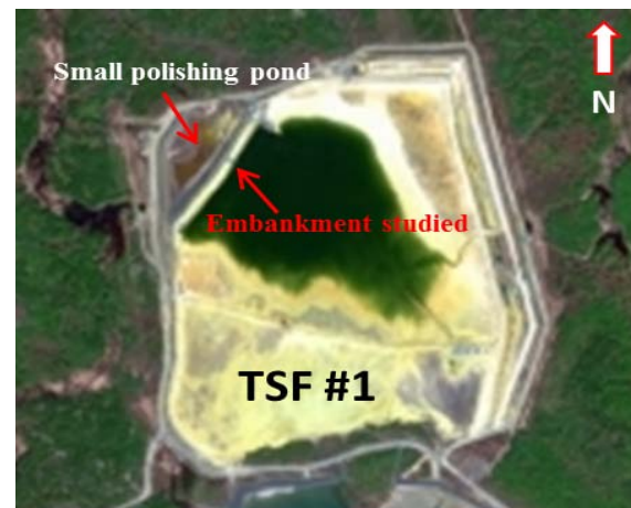
Figure 1: Aerial view of the tailings embankment studied.
