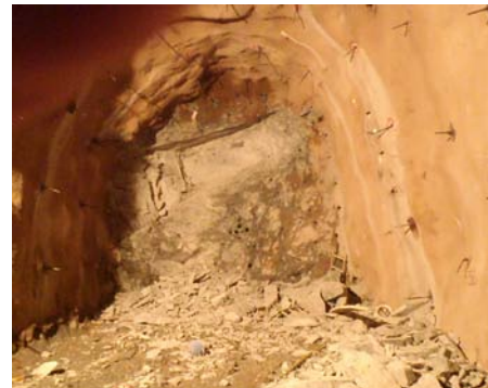
Figure 4: Rockburst at the face excavation in the headrace tunnel.
