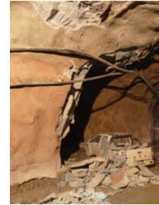
Figure 2: Areas affected by the stress event occurred on 21/03/2012 and a picture of the effects in the by-pass tunnel.
