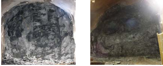
Figure 14: Tunnel face at rockburst events in Headrace tunnel.
