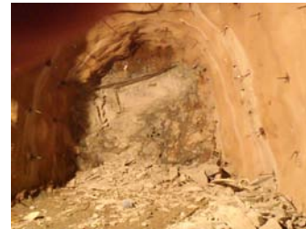
Figure 3: Rockburst at the tunnel face in the Headrace tunnel.
