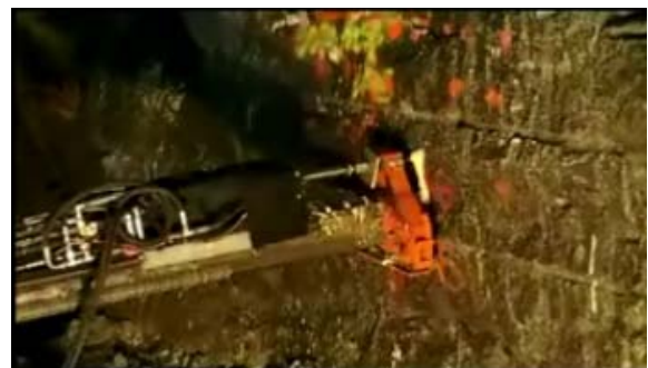
Figure 2: Drilling and injection of pumpable resin using a fully mechanized bolting rig.
