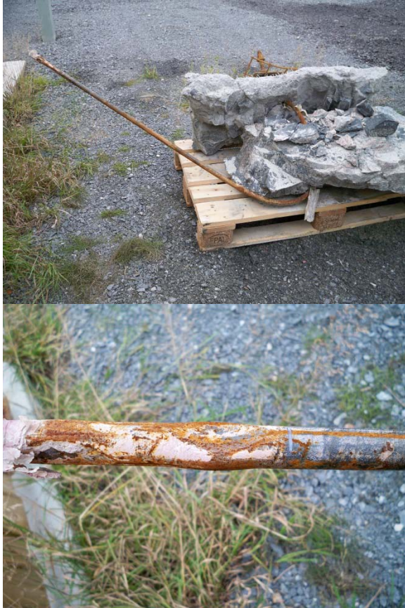
Figure 1: Bolt and rock ejected during a rockburst due to poor encapsulation of the rockbolt in resin.
