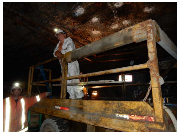
Figure 5: Scissor truck used to install rockbolts in the back of the excavation.
