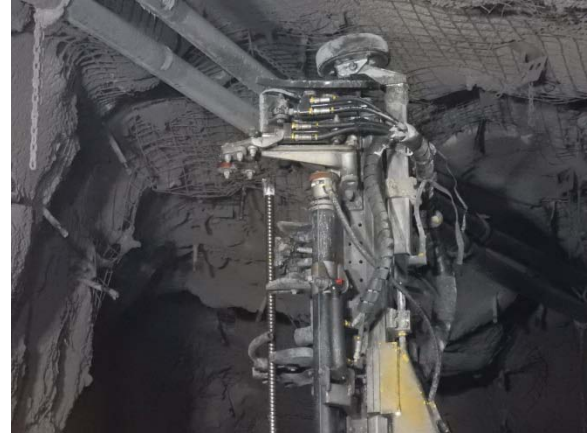
Figure 7: Mechanized bolting rig used to install the Self Drilling rock bolts.
