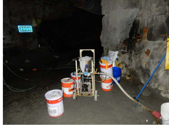
Figure 4: Pump and resin containers used during the test grouting of the D-Bolts.
