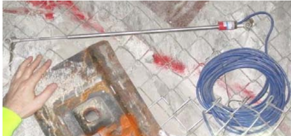
Figure 3: Crackmeter installed across an exposed fault in the wall of a ramp entry at the Lucky Friday Mine.
