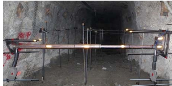
Figure 4: Single-acting closure meter and two earth pressure cells installed in the 5550-11W stope prior to backfilling.
